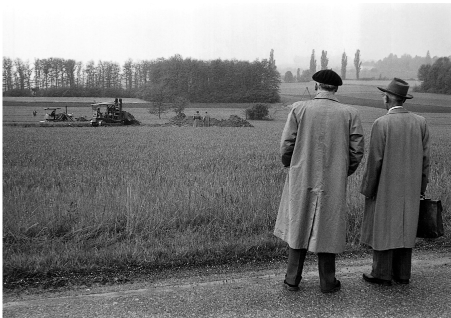
Figure 4.2: The construction of CERN in Meyrin. Taken from [51].
